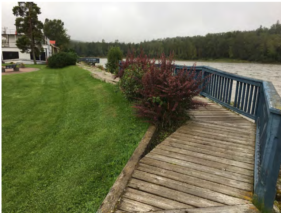
Photograph 5-1: Earthen Dike along Skeena River in Hazelton (August 27, 2020)
